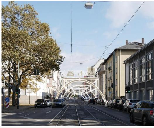
No tree should have to give way to the Frankfurt bridges infrastructure project: Where there are old trees, the bridge section runs over the treetops - with glass inserts in the ground. On narrower roads, almost the entire bridge corpus is made of high-strength trafficable glass, so that it also remains very light under the bridges.
