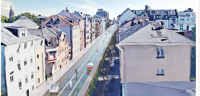
At critical bottlenecks, the bridge is to be designed using highstrength glass that is opaque when ground, but allows daylight and sunlight to pass through almost completely.A similarly polished screen protects the privacy of the adjacent houses and for noise protection, the sides of the bridge between the piers could even be partially glazed down to the ground.
