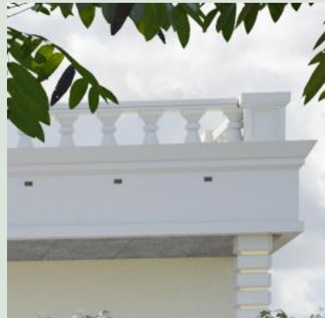
Building blocks in the facade as a roost for bats
