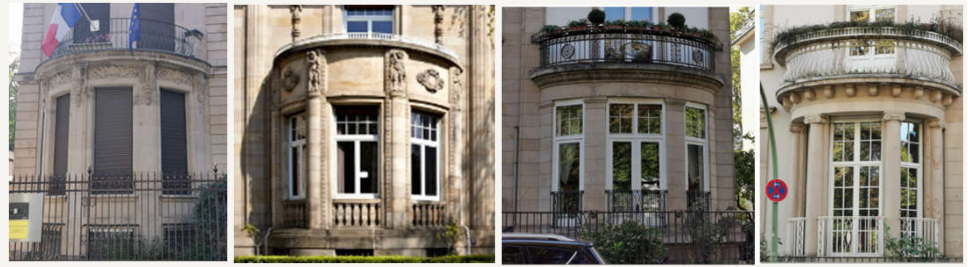
Style models in Frankfurt form the basis. Here: ground floor round bay, partly with balcony
